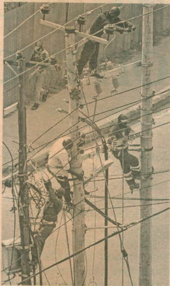
Kenya Power Company technicians at work on Nyerere Avenue, Mombasa. FILE
